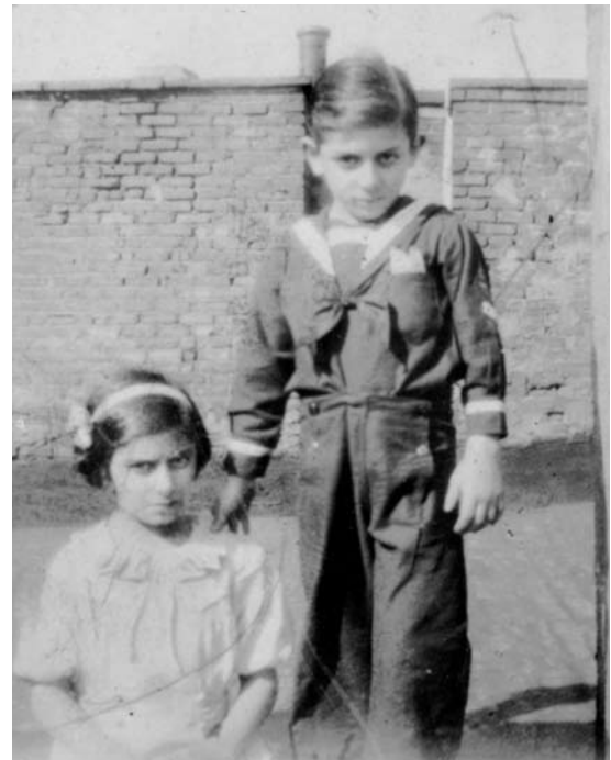
Johnny and Josephine Baldizzi on the roof of 97 Orchard Street, circa 1935.
