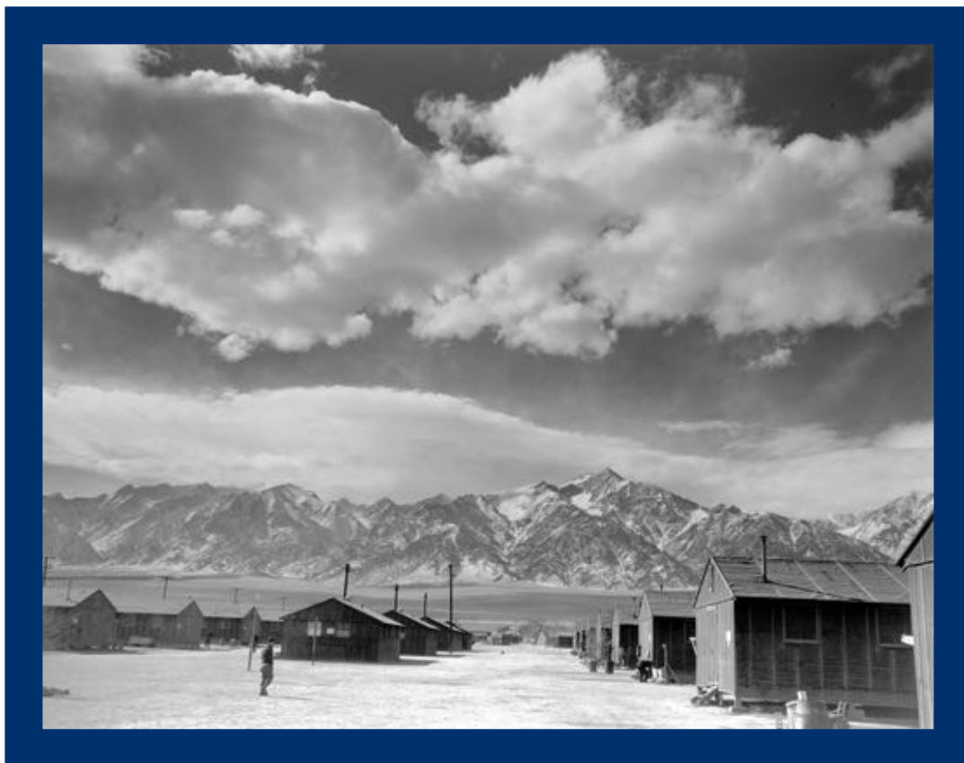
Figure 7. Manzanar Relocation Center, California
