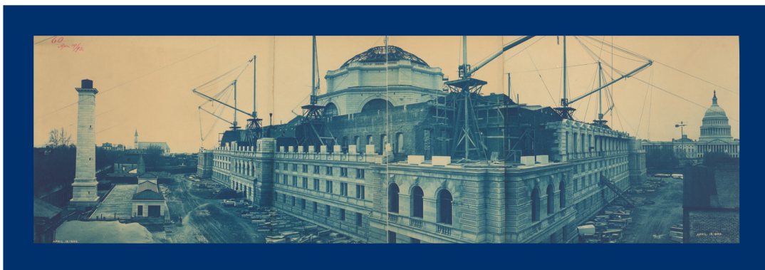
Figure 1. Construction of the Library of Congress, Washington, D.C., April 19, 1893
